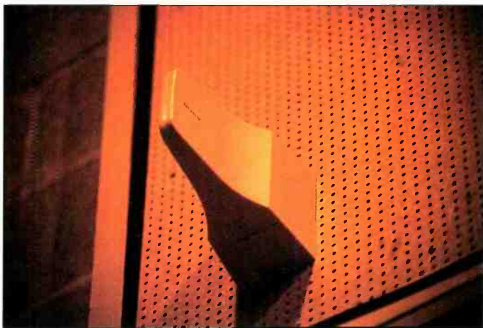
One of a pair of diversity receive antennas for a permanently installed UHF wireless microphone system. The other antenna is mounted on the same studio wall, about 30 feet away.
